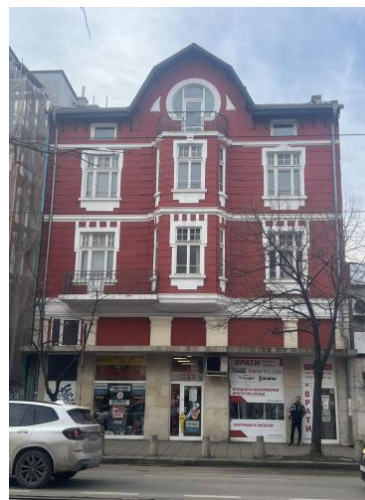
3 Frontal entrance facade2025
