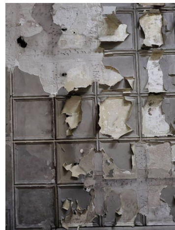
4. Decorative ceiling plaster.
