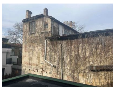
4. Side -facade-2025 (no traces from pre-existin windows)
